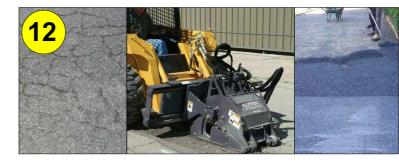
Existiing Path adjacent to the South East boundary is damaged and crazed . It is proposed to remove the top layer of the path with a planer and redress the top surface, as indicated on photos above.
