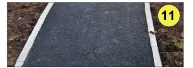
Provide and install new Tarmac path 1500mm wide and edged with concrete pre-cast edging.
